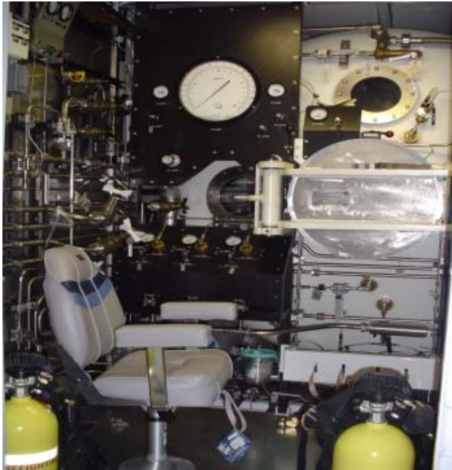
SDS Control Room (Note the Transfer Lock below the viewport)
